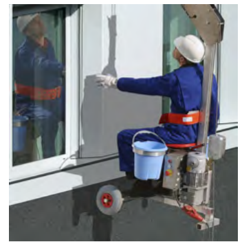
Work seat during repair work.
